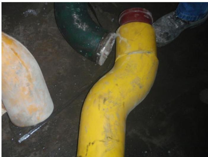
To connect the CDD to the concrete pipe in a simple procedure it is jointed to the concrete pipe with a clamp that can be opened. If the CDD will break it is easy to replace it in this way.
